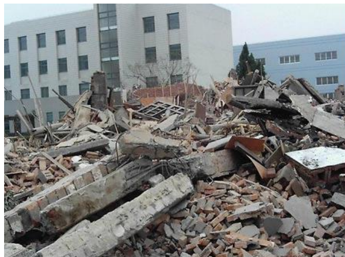
Fig. 1 Demolished construction waste in urban areas
